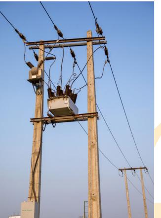
An installed auto-recloser unit for reduction of downtime on tran-Introduction of auto-reclosers for reduction of down-sient faults and to provide selective isolation of fault areas
